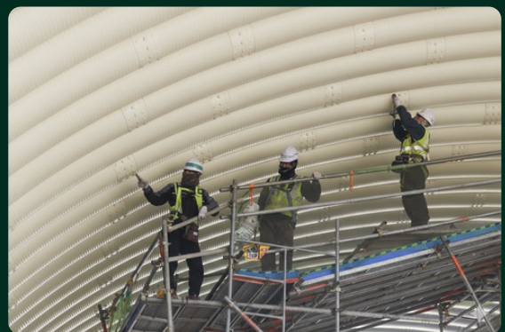
WonderArch Method (Assembly after electro-coating)
