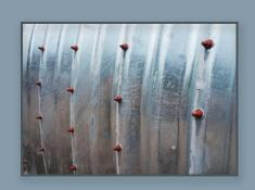
Crosssectional deformation monitoring Corrugated steel plate structures measure the change in cross-sectional shape and size 1 immediately after assembly, 2 during backfilling (including the soil cover section), and 3 immediately after construction is complete.
